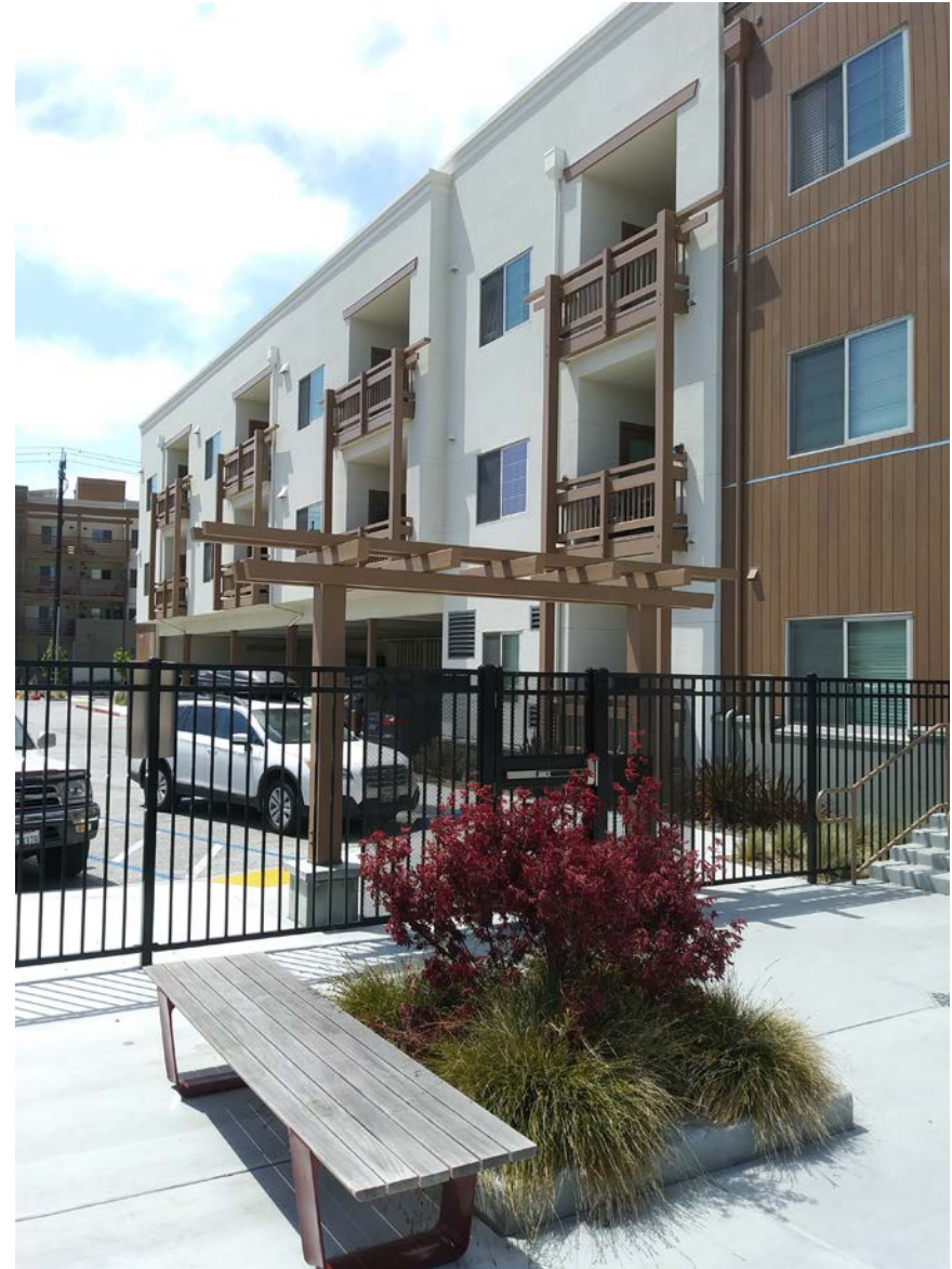
Torii gates included in the architecture of the Dai-Ichi Village multi-family apartment complex.
