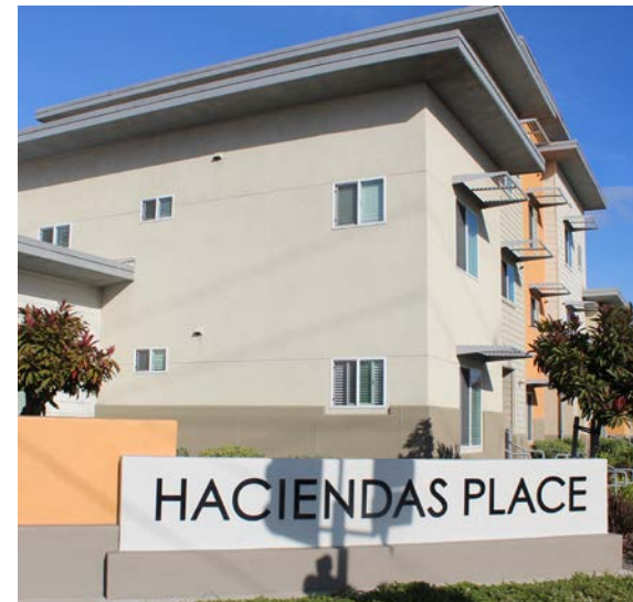
Haciendas Place Phase I and II affordable housing development completed in 2014.
