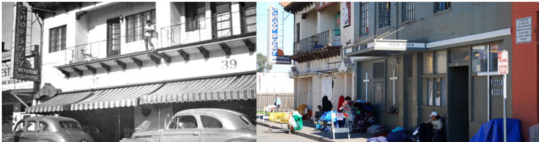
Historic and present day view along Soledad Street and the Chop Suey Republic Cafe Building in Chinatown.
