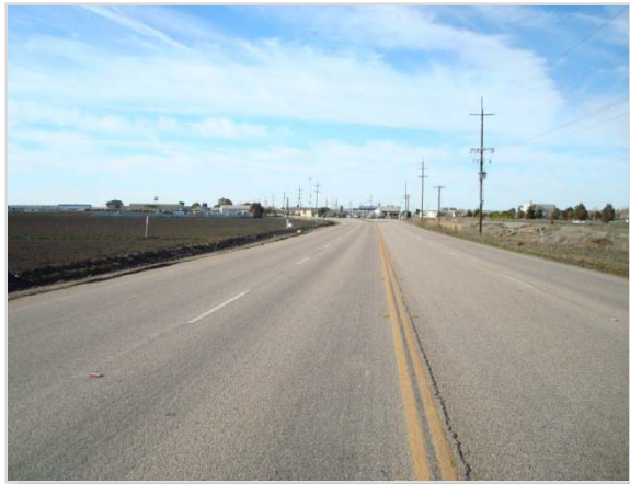
Abbott Street at Project Frontage
