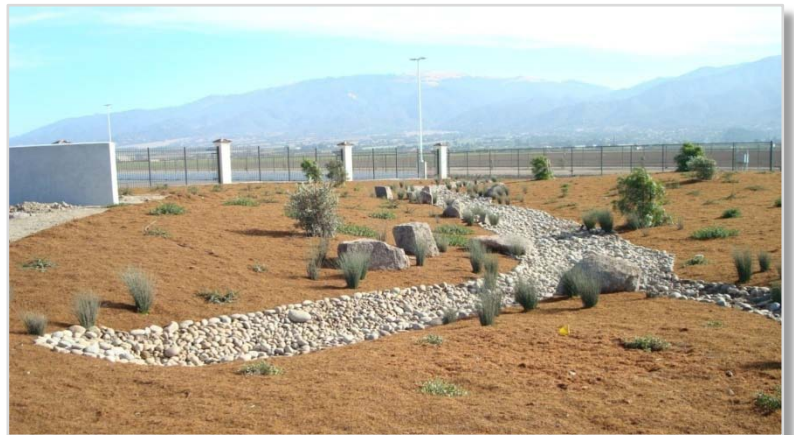
Example of a Post-Construction Stormwater BMP Facility
