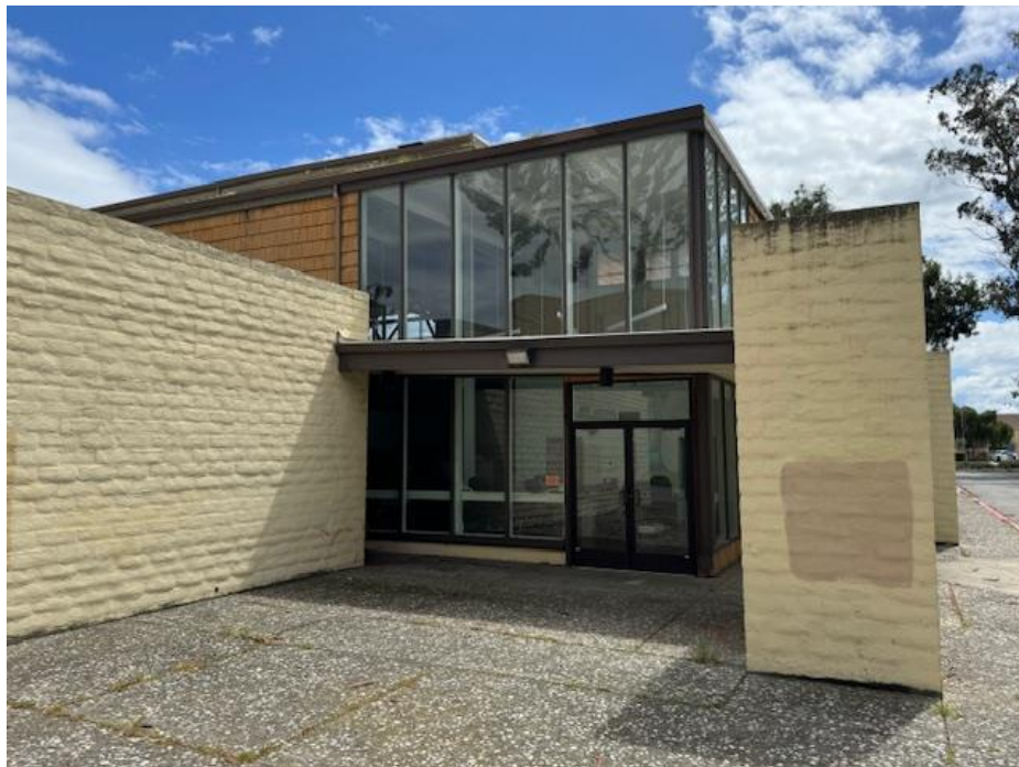
Photograph 4: View looking southwest at the main entrance to the building flanked by CMU walls.
