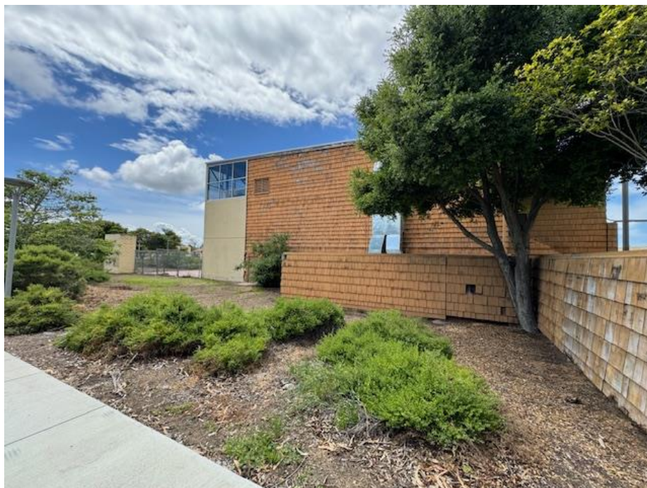
Photograph 12: View looking southwest at the east elevation of the building.
