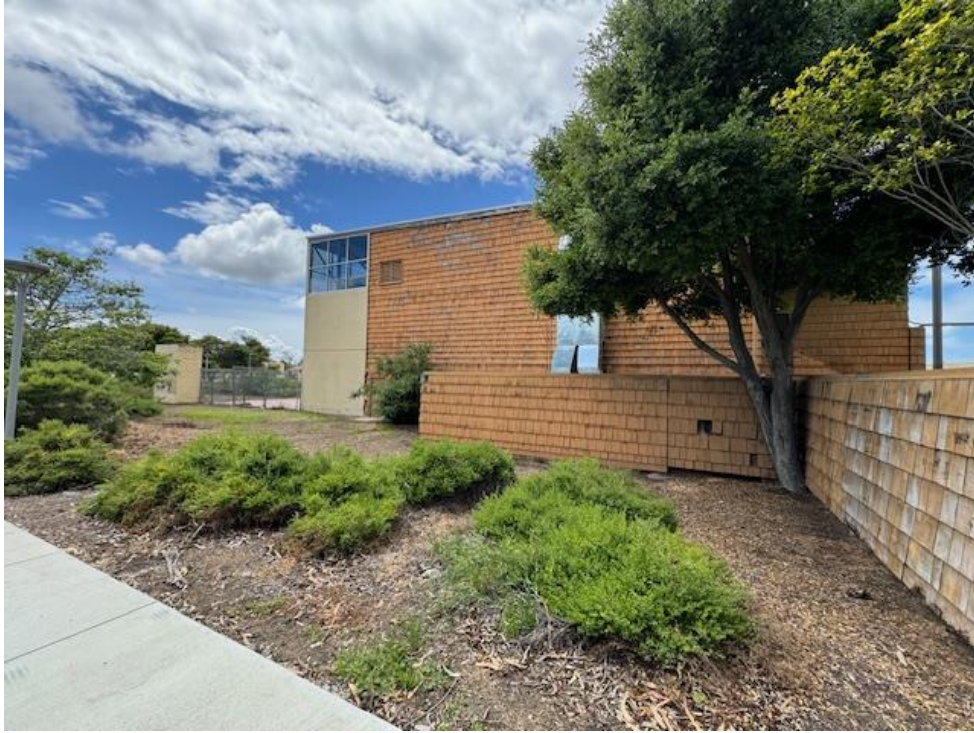
Figure 44: View looking southwest at the east elevation of the building.
