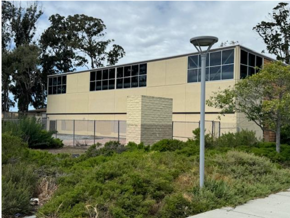
Photograph 9: View looking northwest at the southeast elevation of the building.
