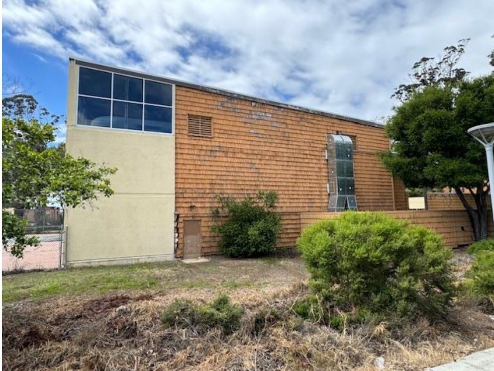
Figure 42: View looking northwest at the east elevation of the building.
