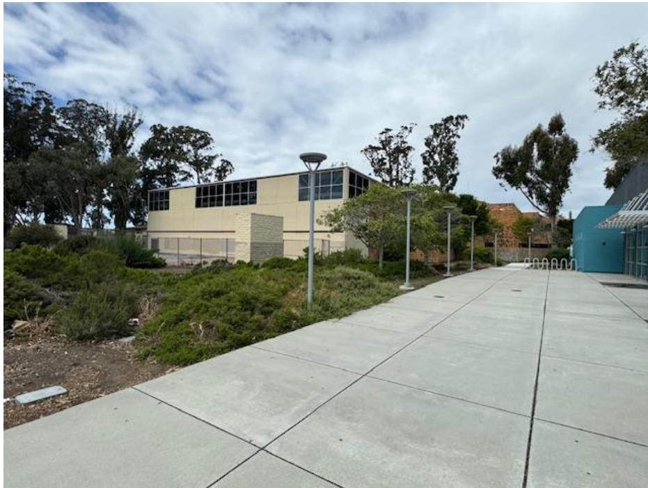
Photograph 8: View looking north at the southeast elevation of the building on the left and on the right the new aquatic center.
