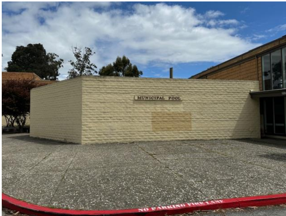
Figure 35: View looking east with the main entrance on the right.
