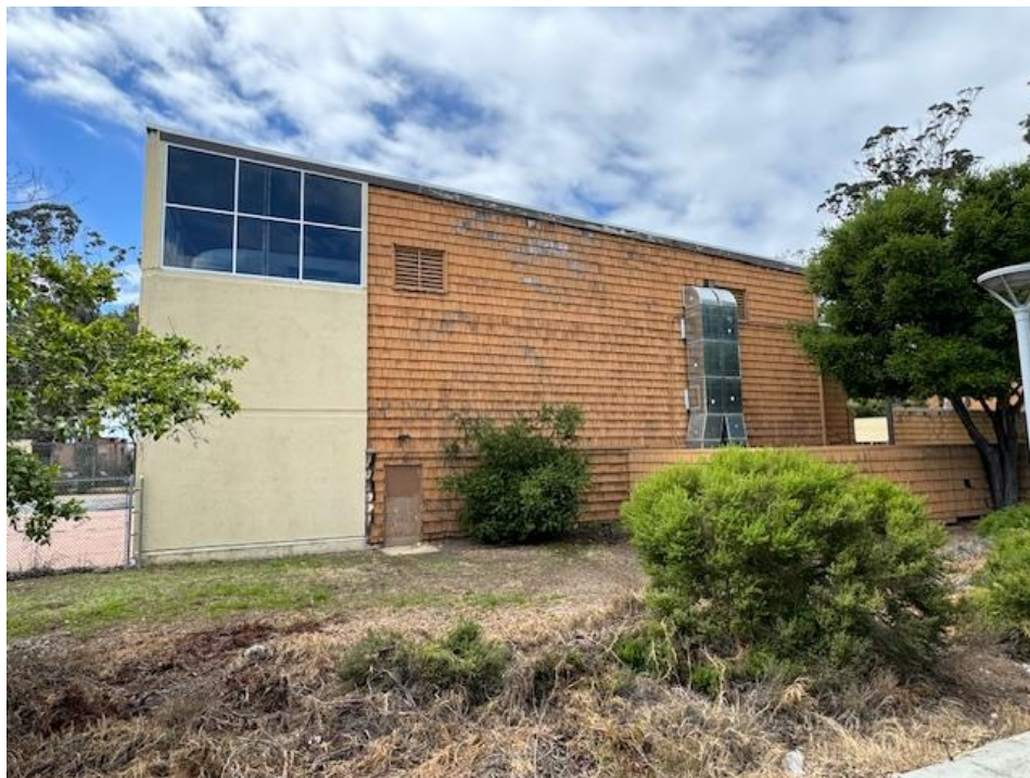
Photograph 10: View looking northwest at the east elevation of the building.
