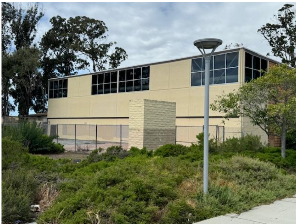
Figure 41: View looking northwest at the southeast elevation of the building.
