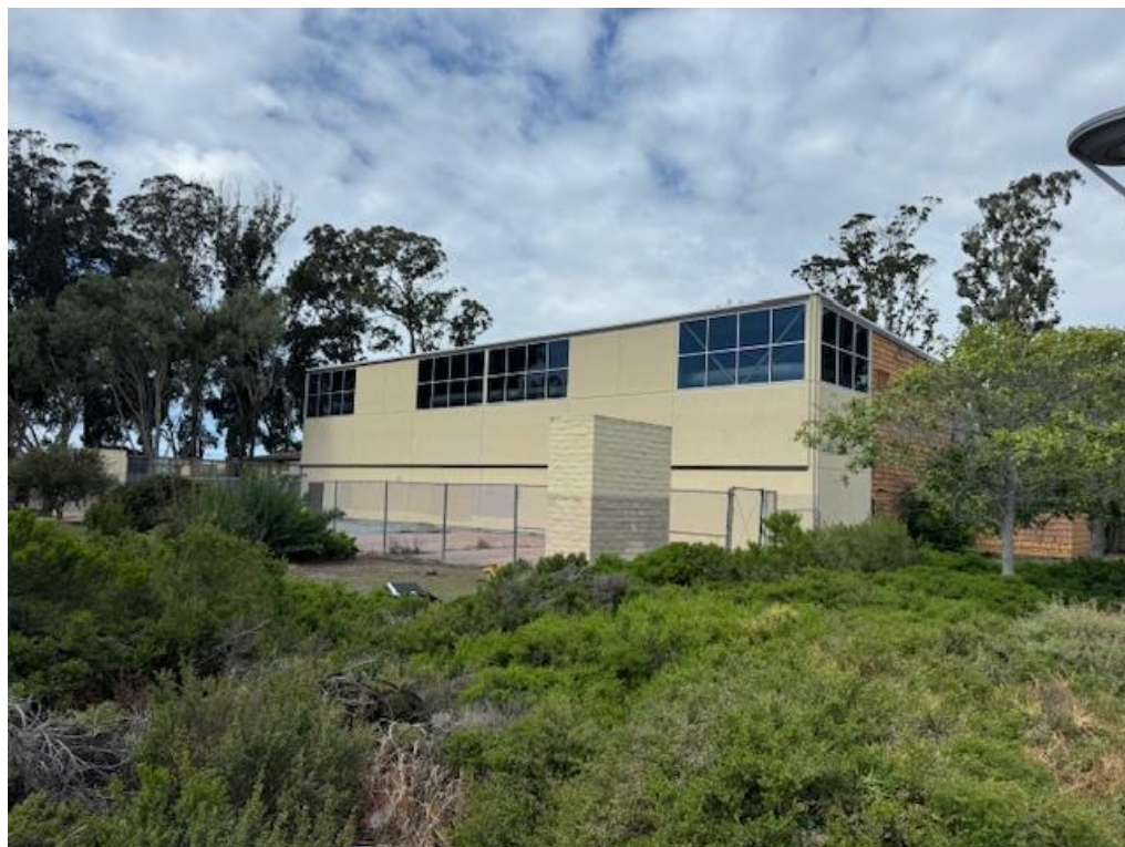
Figure 39: View looking at the south elevation of the building.
