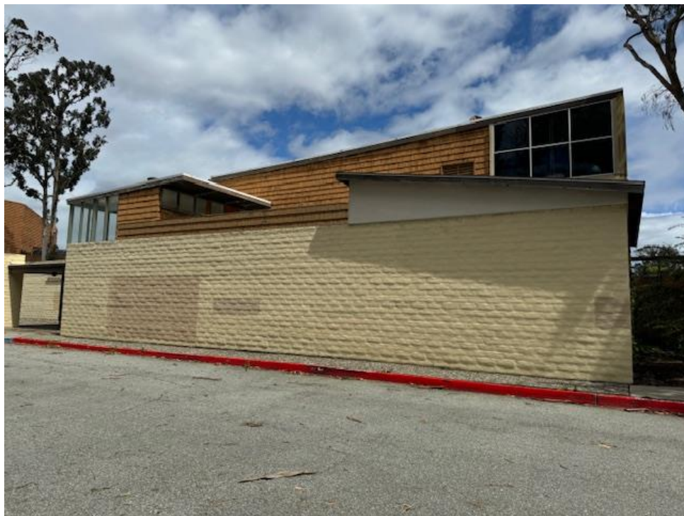
Figure 37: View looking at the east elevation of the building flanked by CMU walls.
