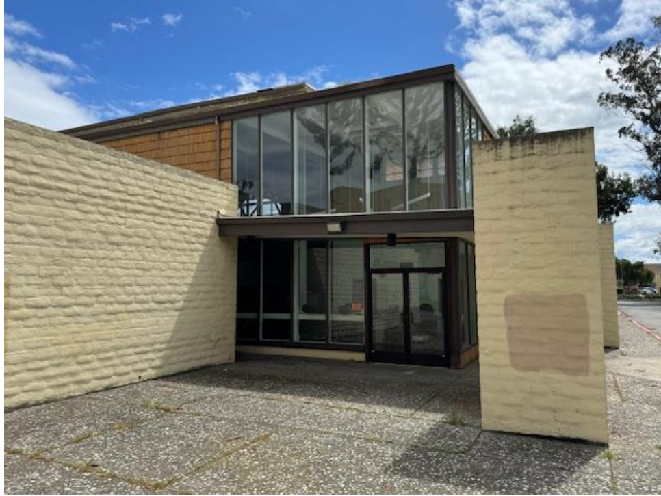
Figure 36: View looking southwest at the main entrance to the building flanked by CMU walls.
