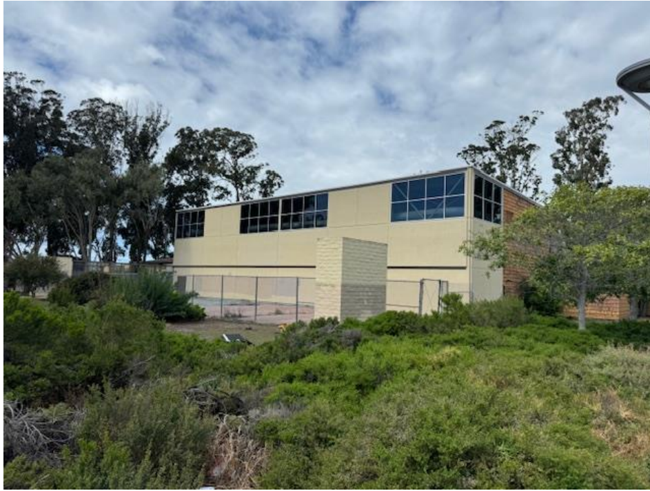
Photograph 7: View looking at the south elevation of the building.
