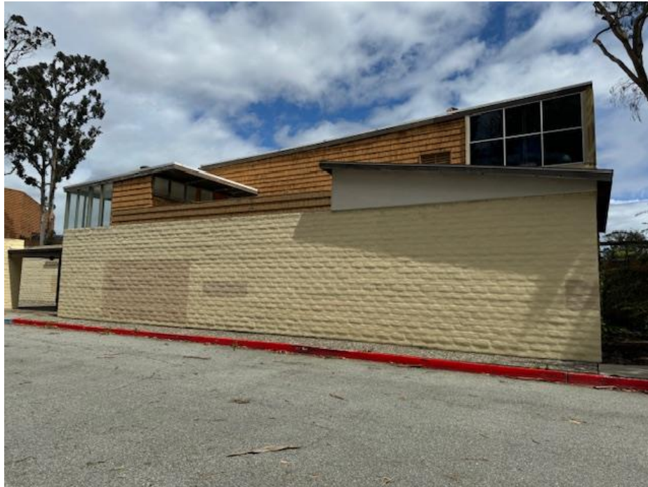
Photograph 5: View looking at the east elevation of the building flanked by CMU walls.
