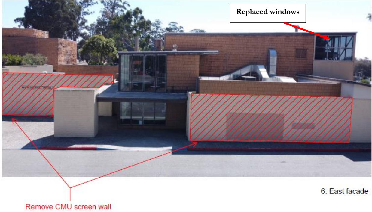
Figure 8: CMU screen wall removal scope of work.
