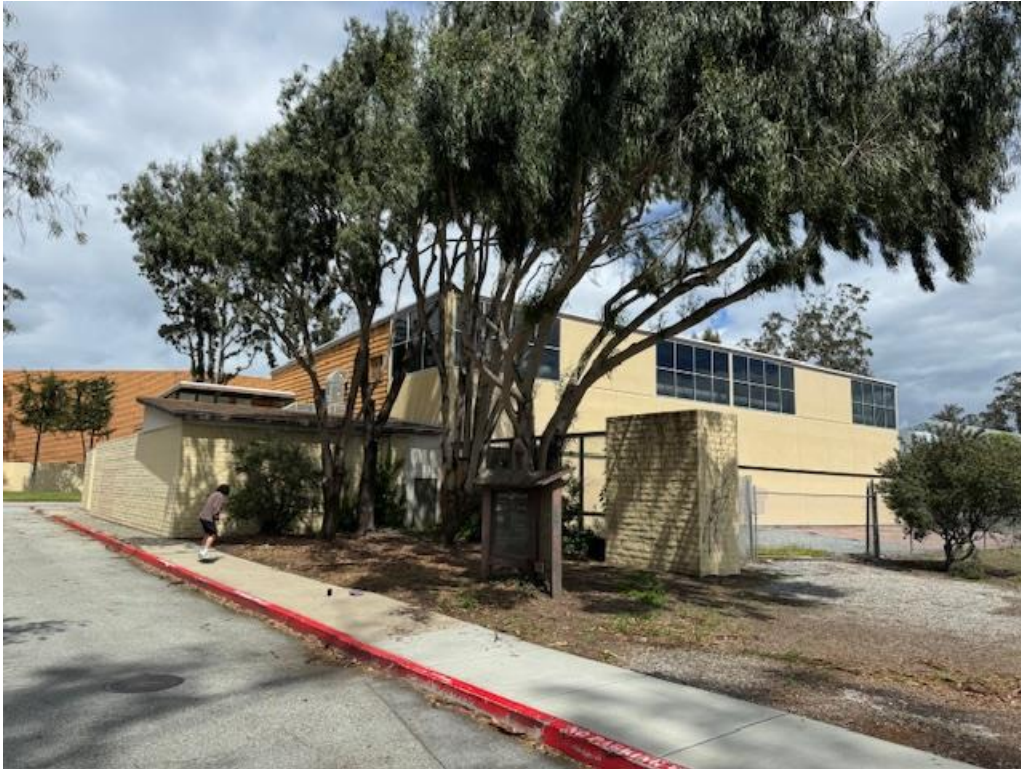
Figure 38: View looking at the southwest elevation of the building.
