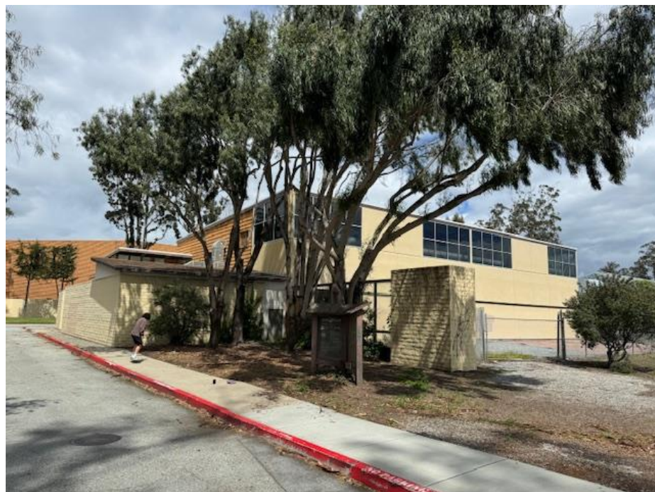
Photograph 6: View looking at the southwest elevation of the building.
