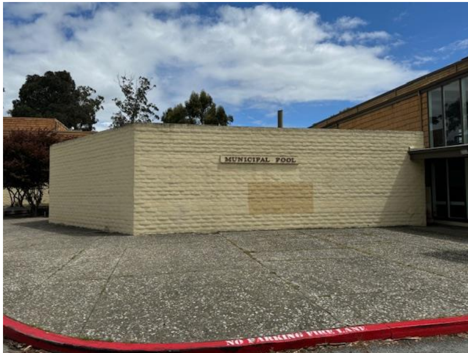
Photograph 3: View looking east with the main entrance on the right.
