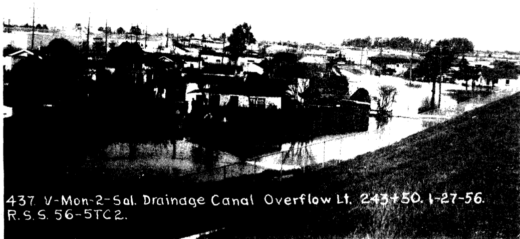
Figure 3. Reclamation Ditch Flooding, Upstream of Carr Lake Near U.S. Highway 101, January 27, 1956
