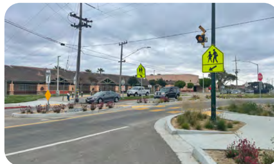
Crosswalk at Bardin Rd and East Alisal St
