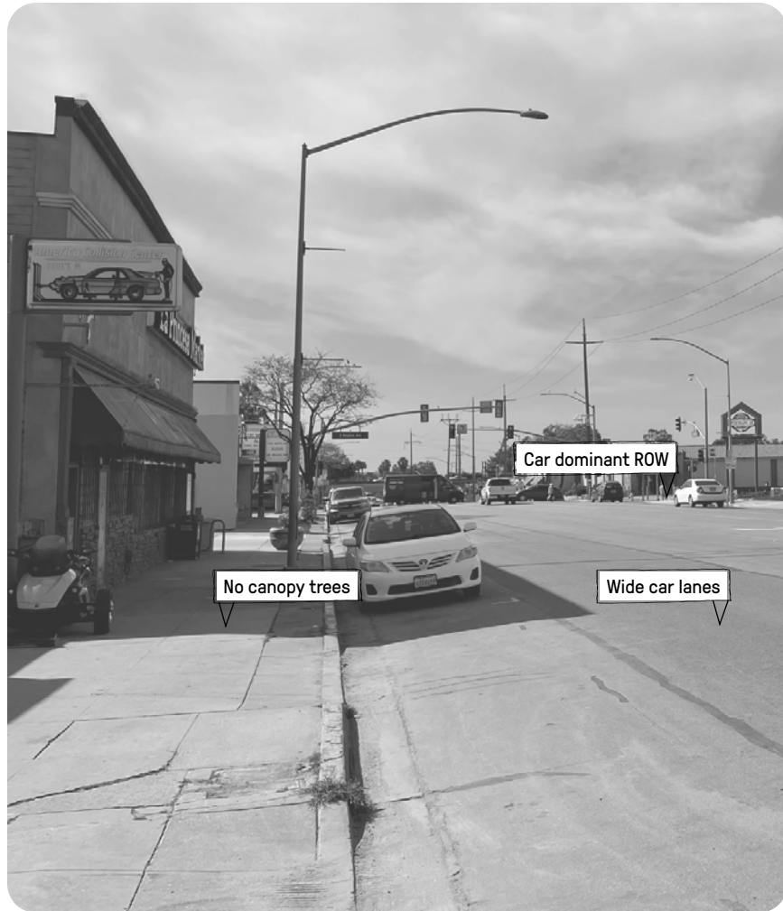
Typology 1. Typical existing road condition at La Princesa Market in East Alisal St
