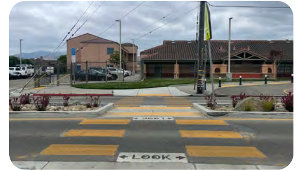
Crosswalk at Bardin Rd and East Alisal St
